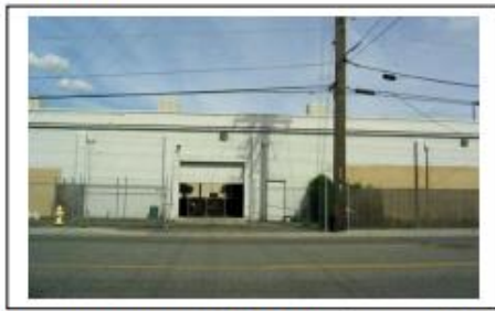
No screening on the backside facing public street.
